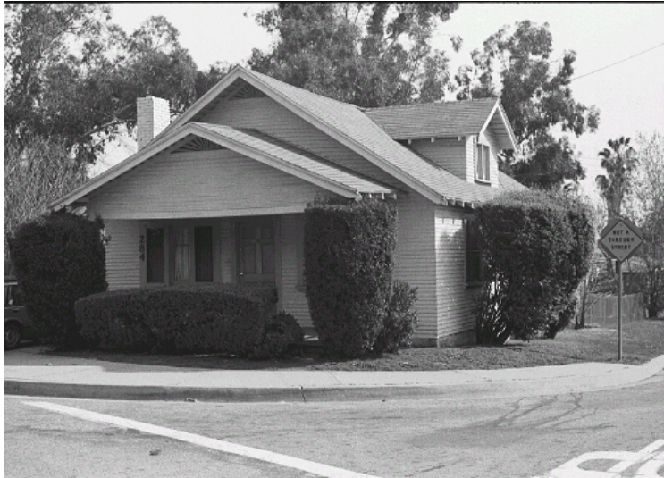
Original survey photo (ca. 1990)
