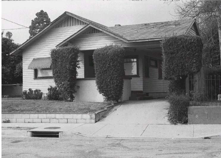
Original survey photo (ca. 1990)
