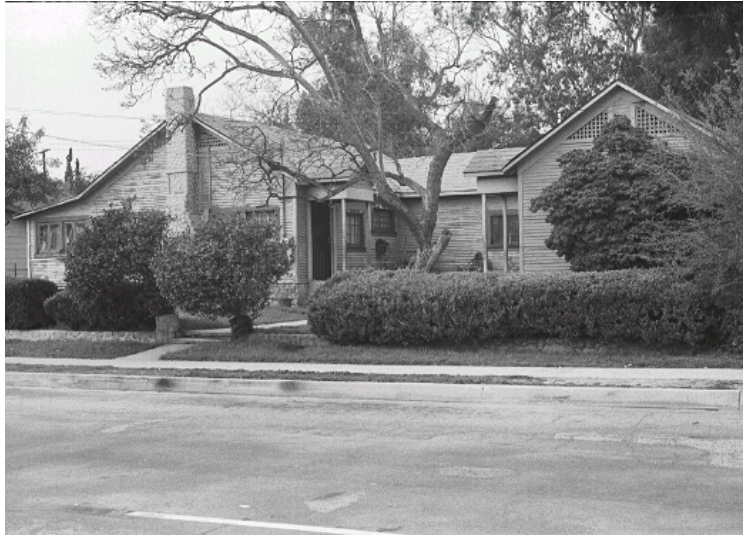
Original survey photo (ca. 1990)
