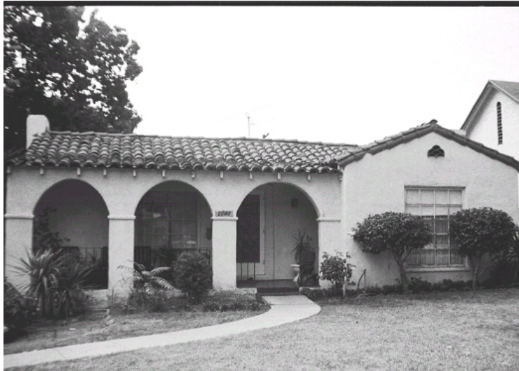
Original survey photo (ca. 1990)
