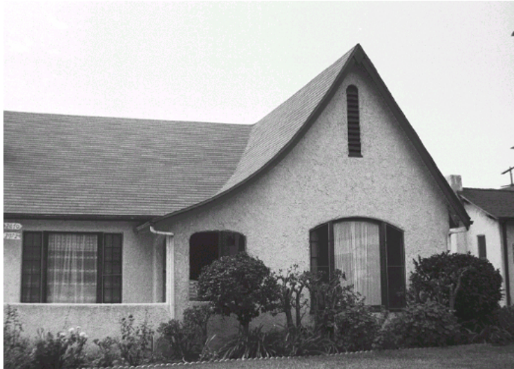
Original survey photo (ca. 1990)
