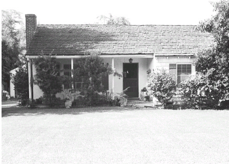
Original survey photo (ca. 1990)
