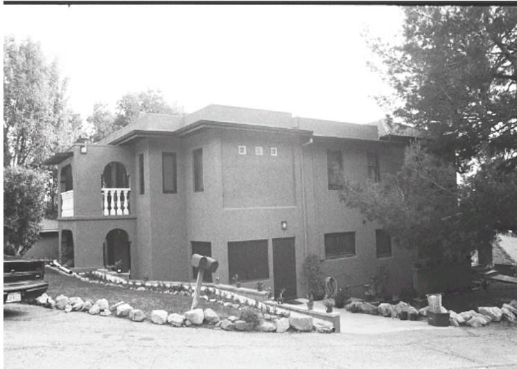
Original survey photo (ca. 1990)
