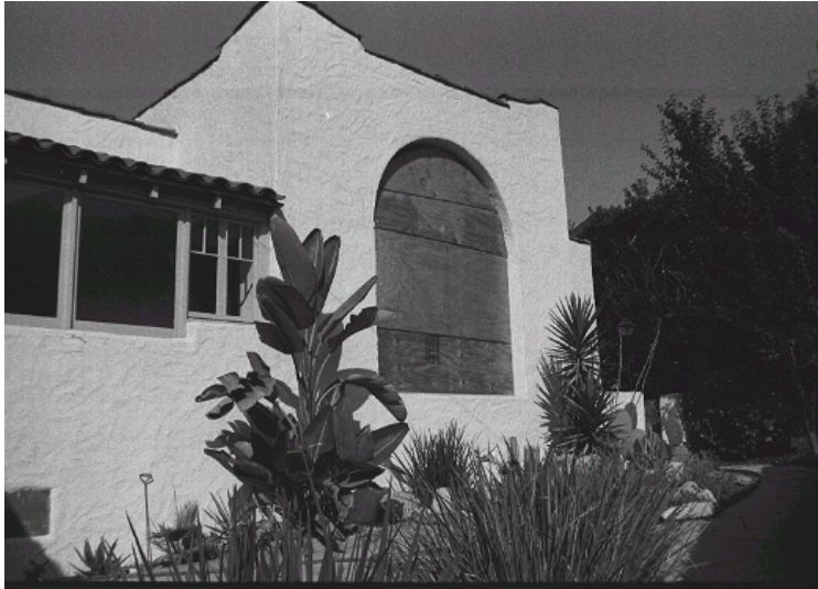
Original survey photo (ca. 1990)
