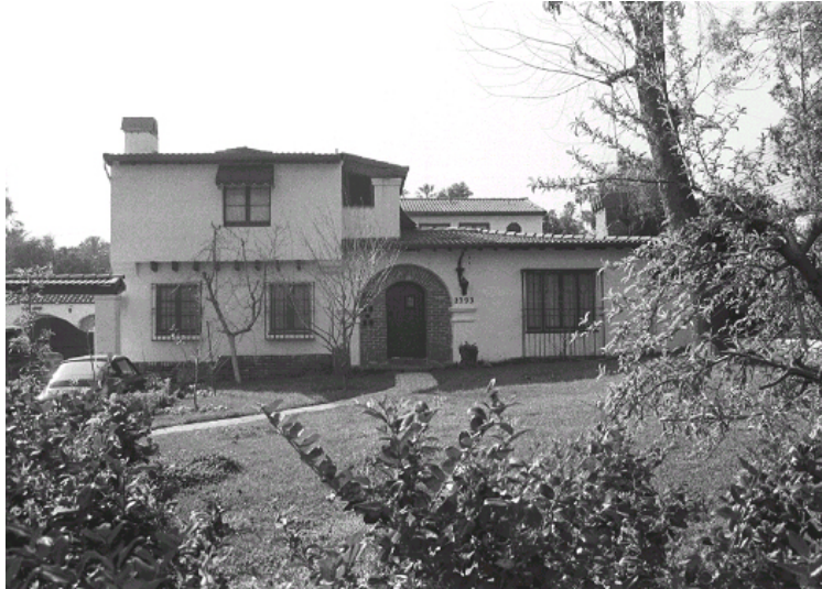
Original survey photo (ca. 1930)
