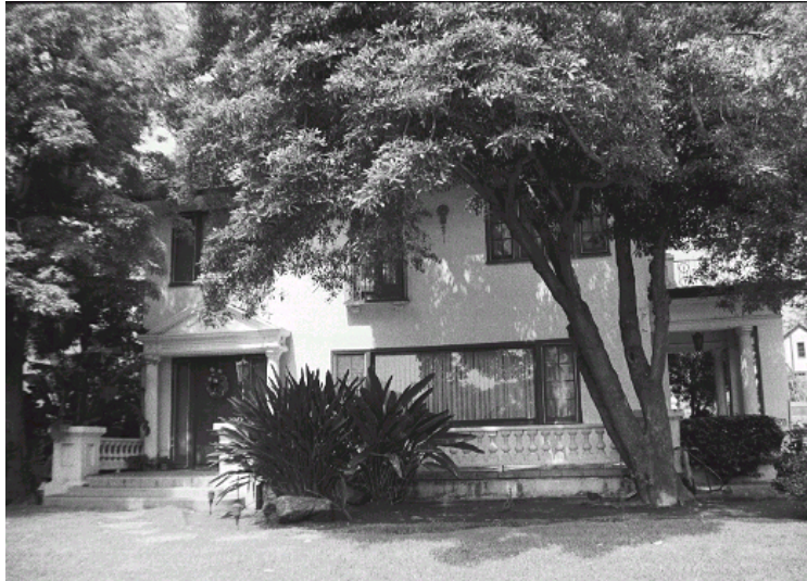
Original survey photo (ca. 1990)
