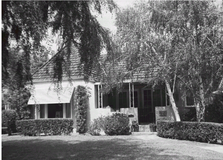
Original survey photo (ca. 1990)
