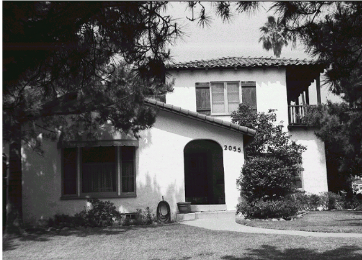
Original survey photo (ca. 1990)
