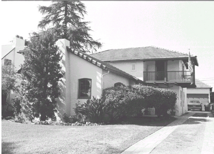
Original survey photo (ca. 1990)
