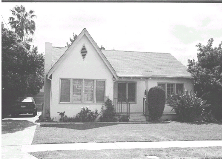
Original survey photo (ca. 1990)
