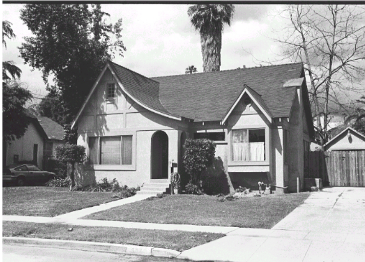
Original survey photo (ca. 1990)
