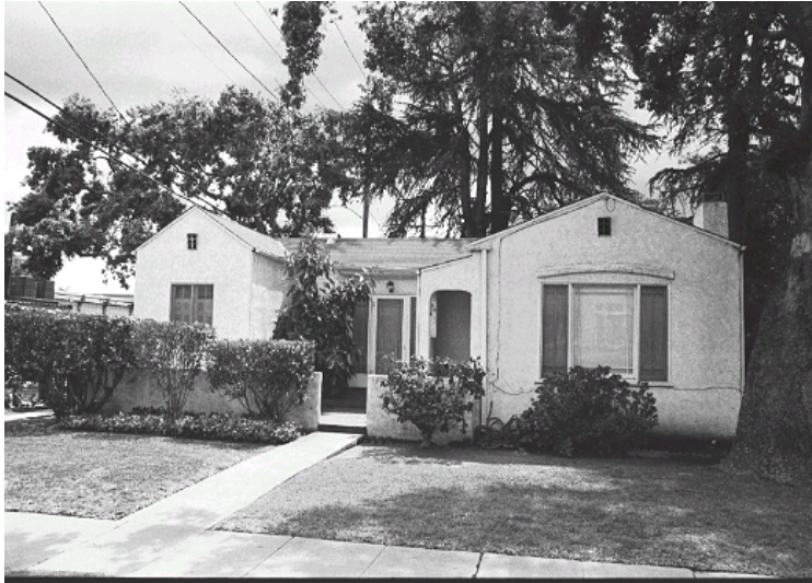
Original survey photo (ca. 1990)
