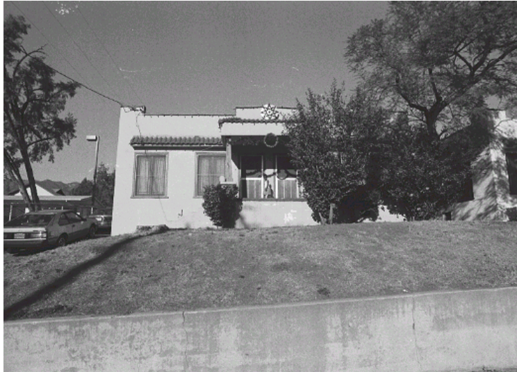
Original survey photo (ca. 1990)
