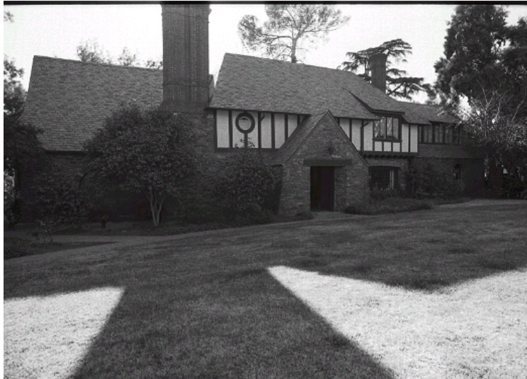
Original survey photo (ca. 1990)
