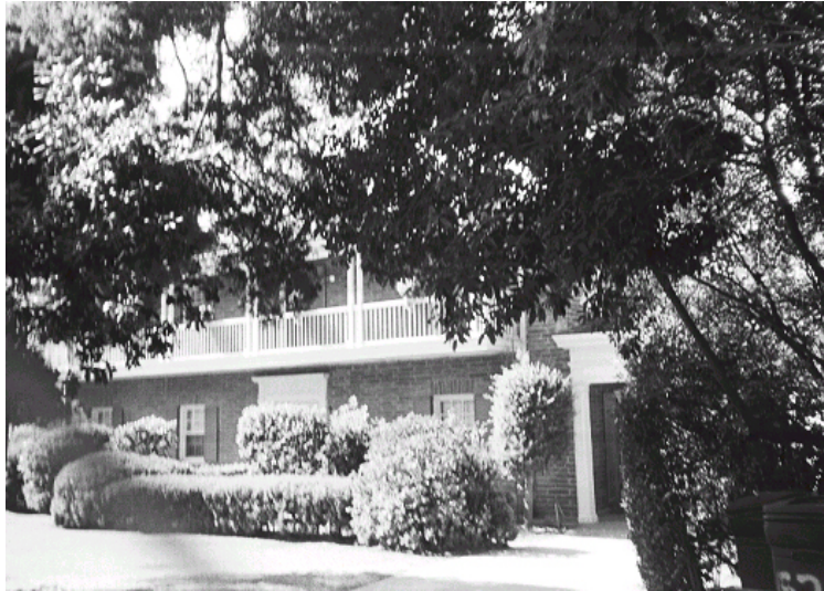
Original survey photo (ca. 1990)
