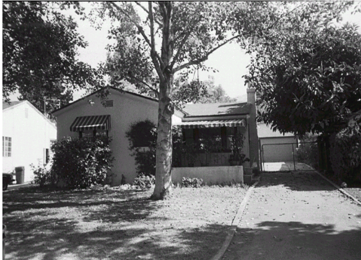
Original survey photo (ca. 1990)
