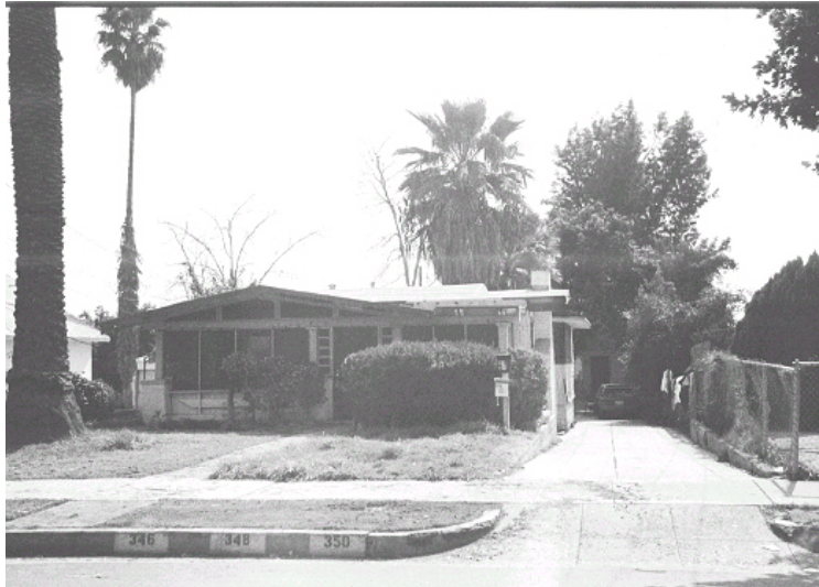
Original survey photo (ca. 1990)
