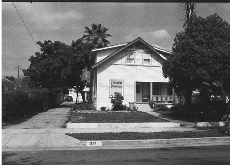
Original survey photo (ca. 1990)
