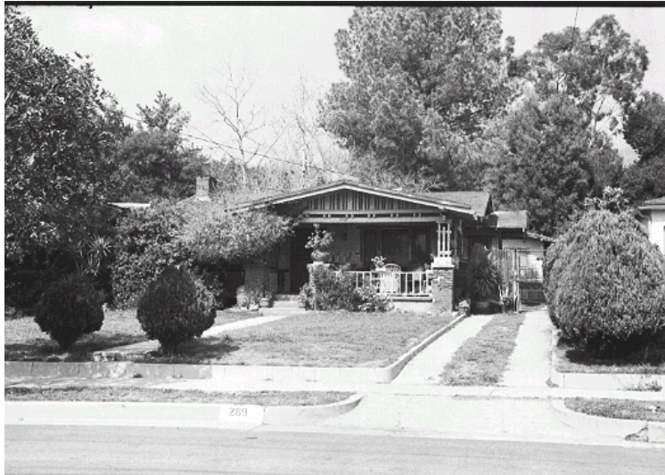
Original survey photo (ca. 1990)
