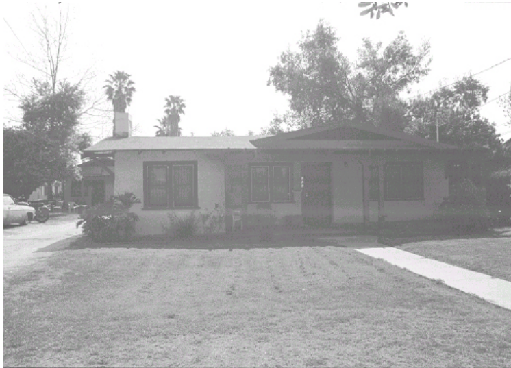
Original survey photo (ca. 1990)
