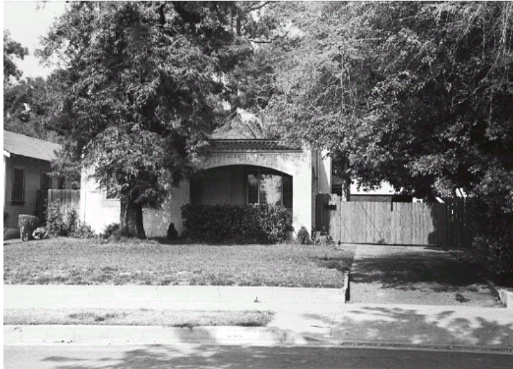
Original survey photo (ca. 1990)
